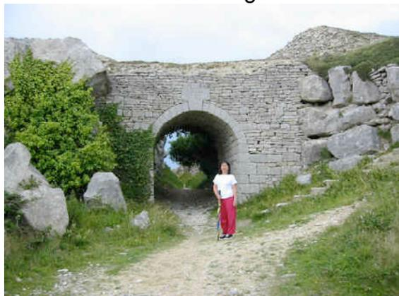
Lano's Bridge was built in the mid-1800s to carry a high level tramway taking spoil to the cliff edge with a low level tramway going through the arch taking stone to the Merchants' Railway. <sup>1</sup> We do not have any information as to whether our Richard Lano was involved in the construction of this bridge but it does
